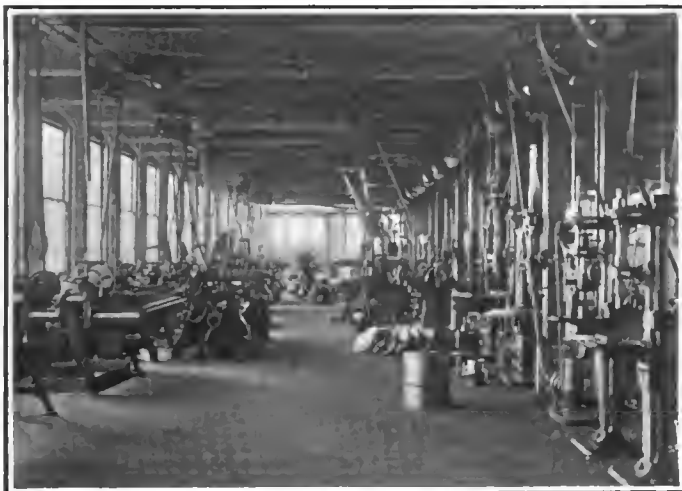
MACHINE DEPARTMENT ON SOUTH HALF OF MAIN FLOOR.
